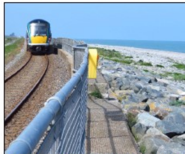
Proximity of railway line to shore at Six Mile Point.
