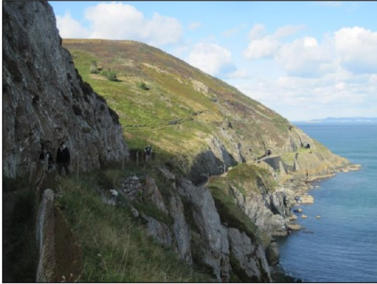
Looking north along the cliff path, with footpath above the railway line.
