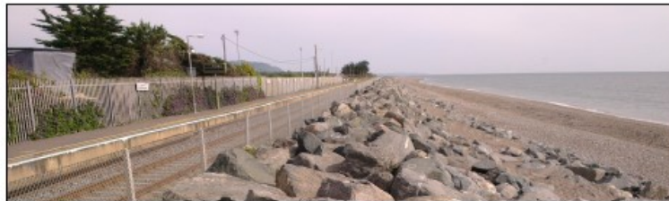
Coastal defences at Kilcoole Railway Station, looking north.
