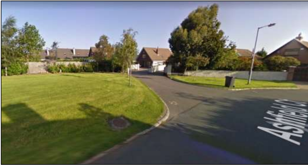
Figure 1 Permitted backland development in Bray also with access across open space from a curved portion of roadway at a depth of up to 14 metres, where no right of way existed.
