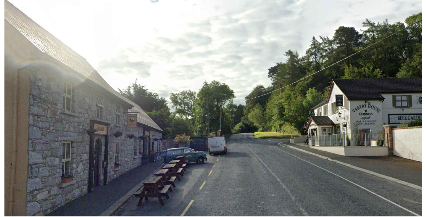
SITE PHOTO VIEW TAKEN FROM BYRNE & WOODS BAR & RESTAURANT LOOKING EAST ALONG R764
