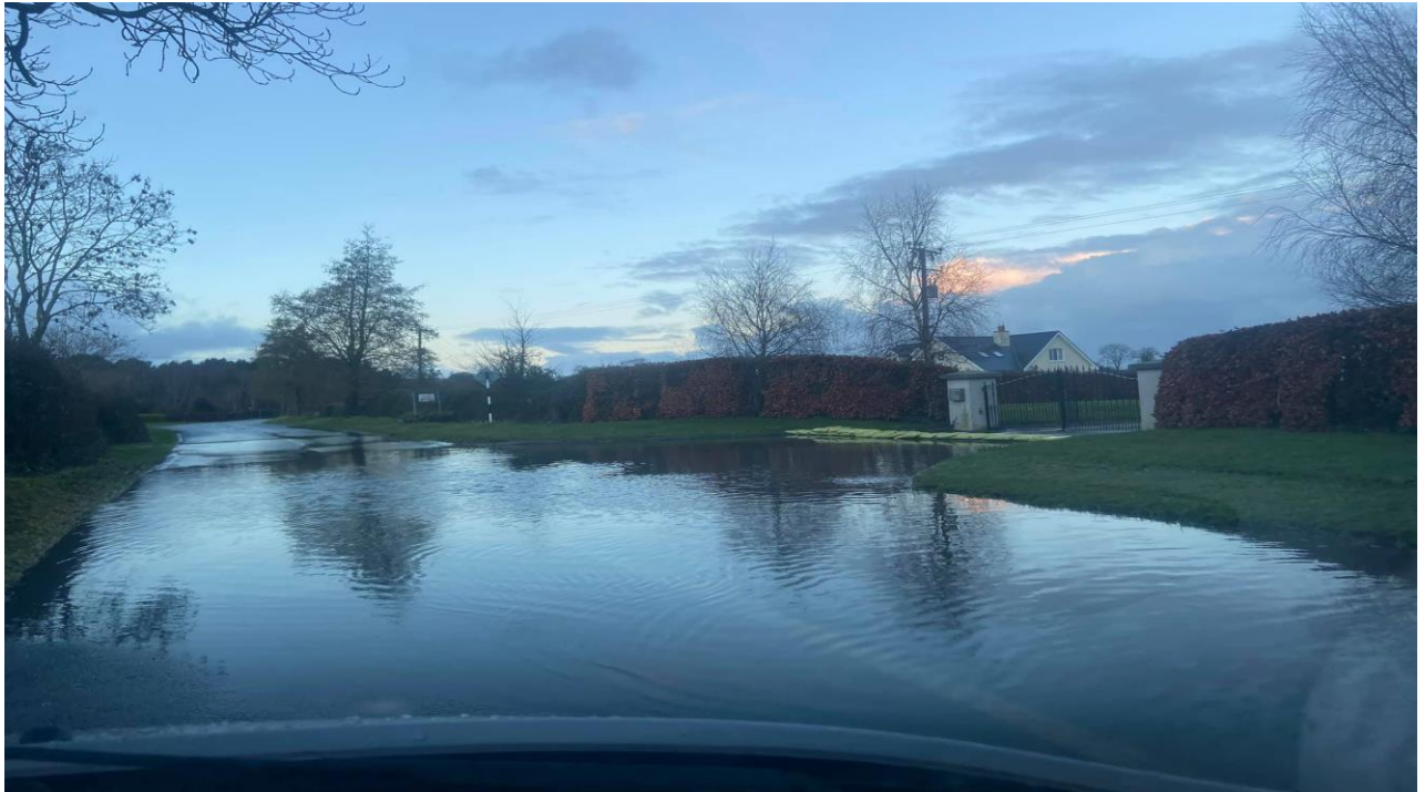
Flooding on R761 north of village in February 2021.
