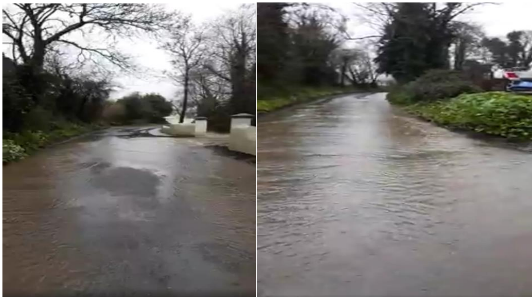
Flooding on Sea Road between Hunters' Leap and the boat repair yard in February 2021.
