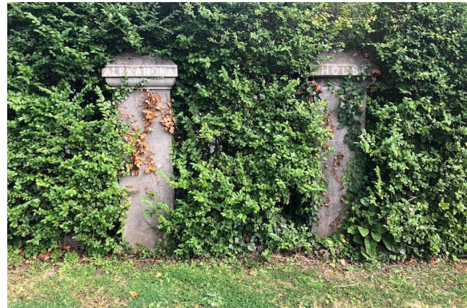
Fig. 28: View of gate posts with pyramidal cappings along Somerby Road left in place.
