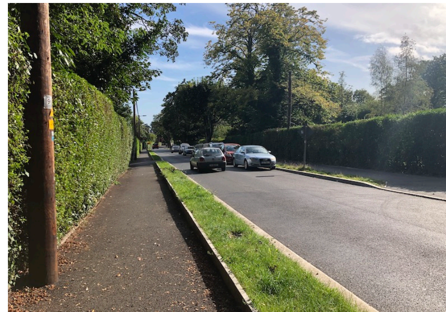
Fig. 34: View recent works to footpath to calm traffic along St Vincent Road.
