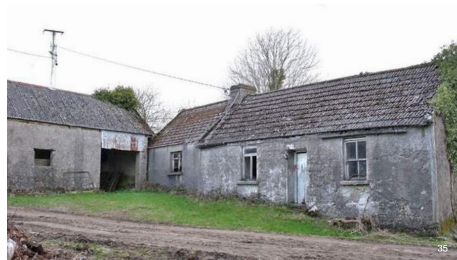
Restoration potential of cottage and outbuildings. Tinahely, County Wicklow.
