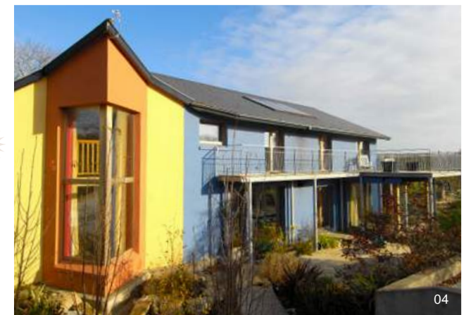
Passive design angled towards the sun with large openings to maximise solar gain.
