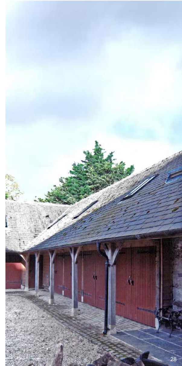
Dutch barn outbuilding conversion. County Wicklow.
